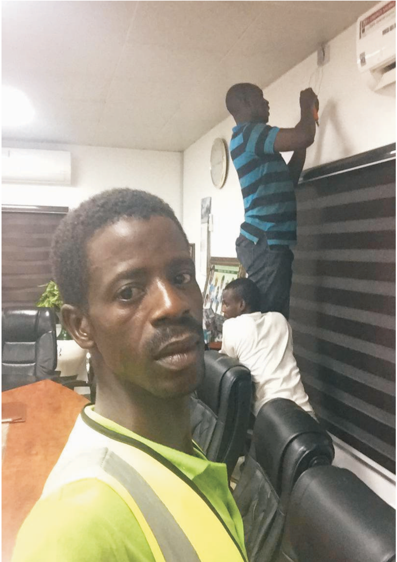
INSTALLATION OF OPTICAL FIBRE
